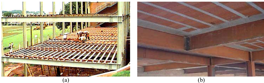
Figure 2 - Execution of a precast ribbed slab in a steel structure building. (David, 2007)
