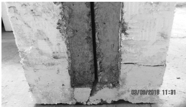
(c) Slab 1 – TREL-2
