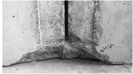
(b) Slab 2 – MAC-01
