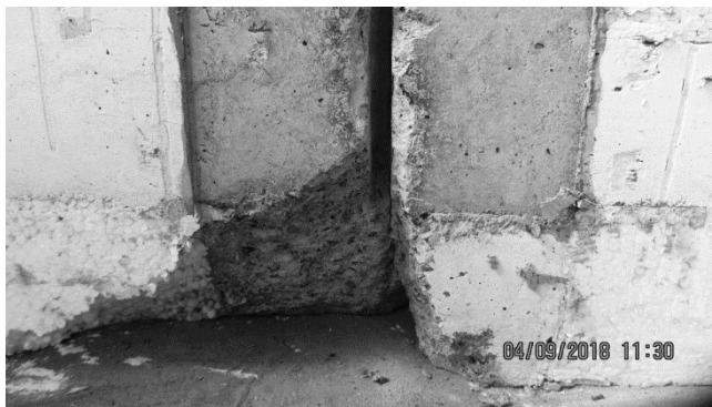
(e) Slab 1 – TREL-3
