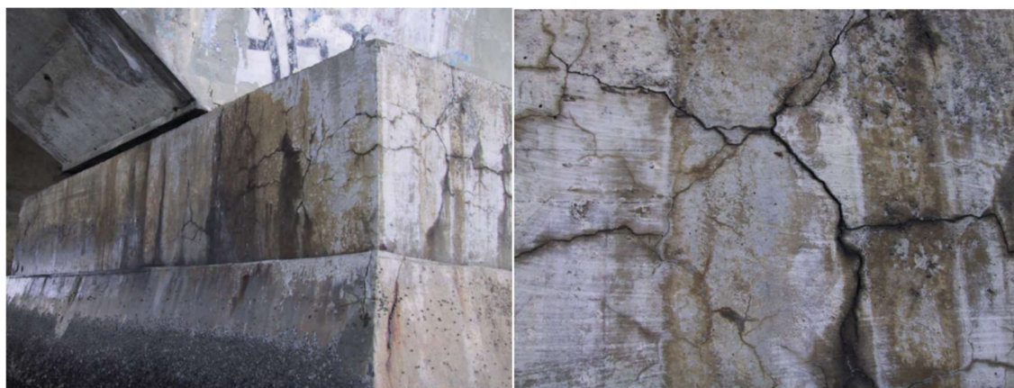
Figure 1 – Deterioration signs at Paulo Guerra Bridge, Recife-PE
