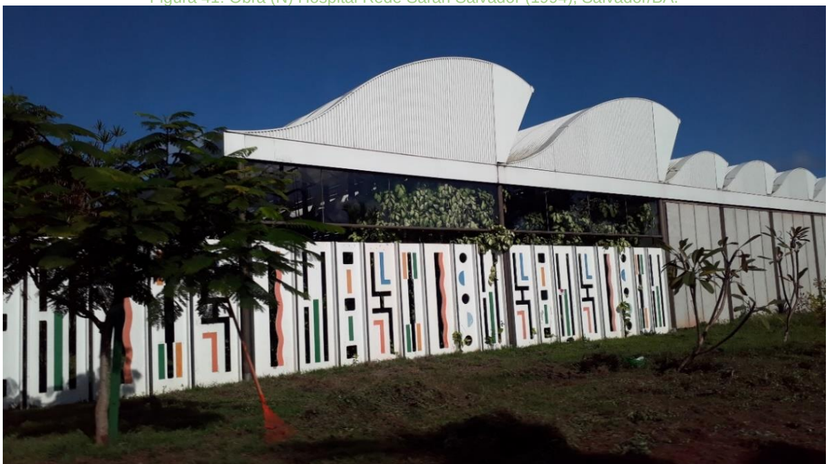
Figura 41: Obra (N) Hospital Rede Sarah Salvador (1994), Salvador/BA.
