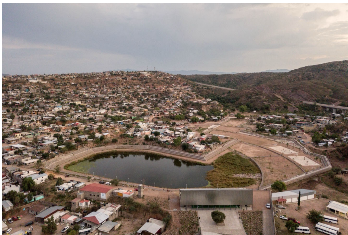
FIGURA 36 - COLOSIO EMBANKMENT DAM
