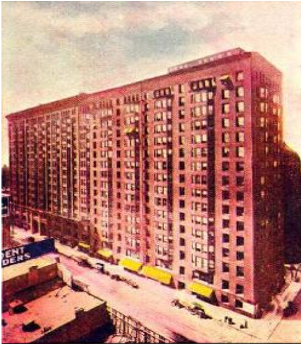
FIGURA 02: Monadnock Building, Chicago-EUA
